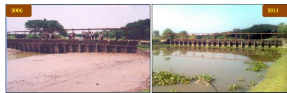
Photo 3: Revival of Hari River near Bhabodah regulator in between 2006-2011 (Source: Paul et al. , 2013)
