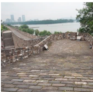
Fig. 1 Overview of City Wall
