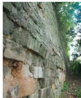
Fig. 6 Extrusion of bricks
