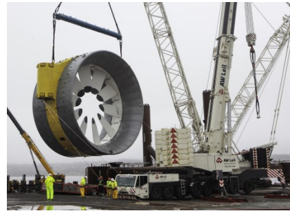
Figure 4 – Assembly of OpenHydro turbine ©OpenHydro
