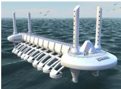
Figure 63 – WEC with UHPFRC. ©Wave Star Energy
