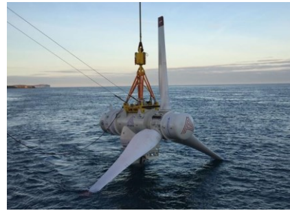
Figure 2 – Andritz Hydro- Hammerfest turbine installed at Meygen, ©Meygen
