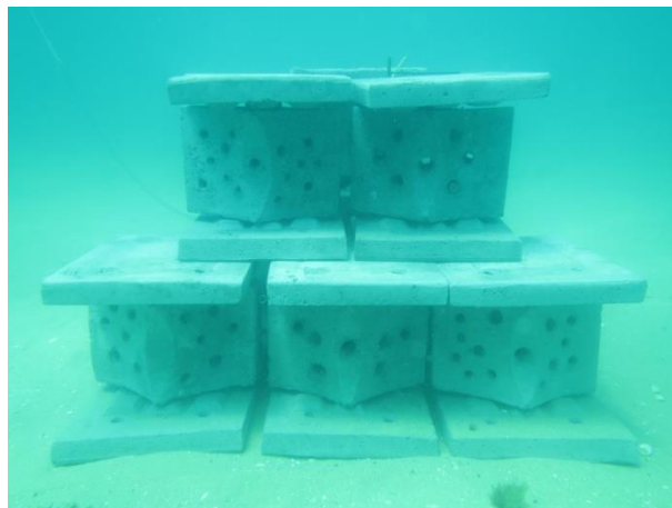
Fig. 3.2 New design artificial reef. a. Lid b. Central piece c. One assembled reef.
