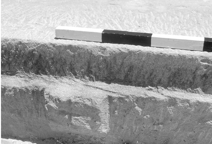
Fig. 13.24. Cypriot ashlar block with mason's mark on lifting boss from Building X, Kalavassos-Ayios Dhimitrios, Late Cypriot IIC, thirteenth century BCE (photograph by L. A. Hitchcock).
