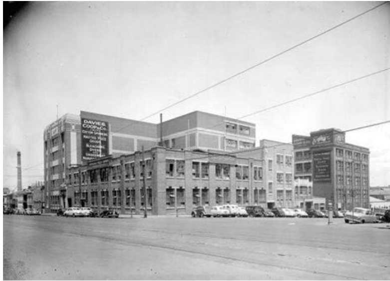
Figure 9.6 The Davies Coop building, which became Lincoln House. 111
