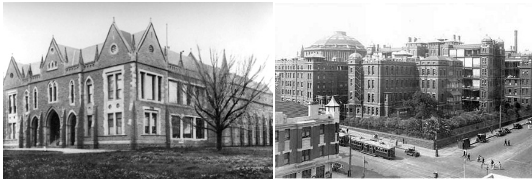
Figure 6.2 The Medical School (left) and the Melbourne Hospital (right). 12
