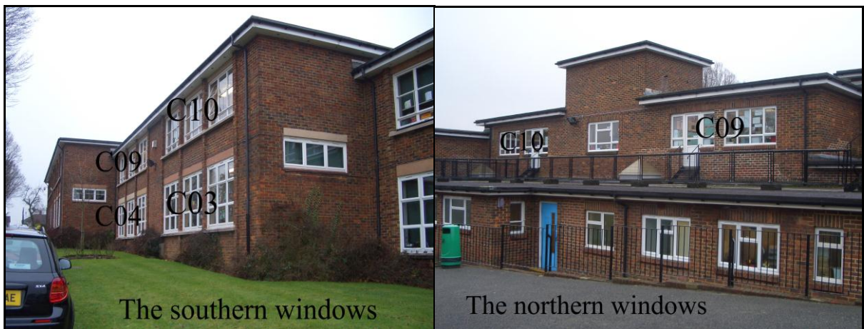
Figure 3.3 The southern and northern windows of the classrooms
