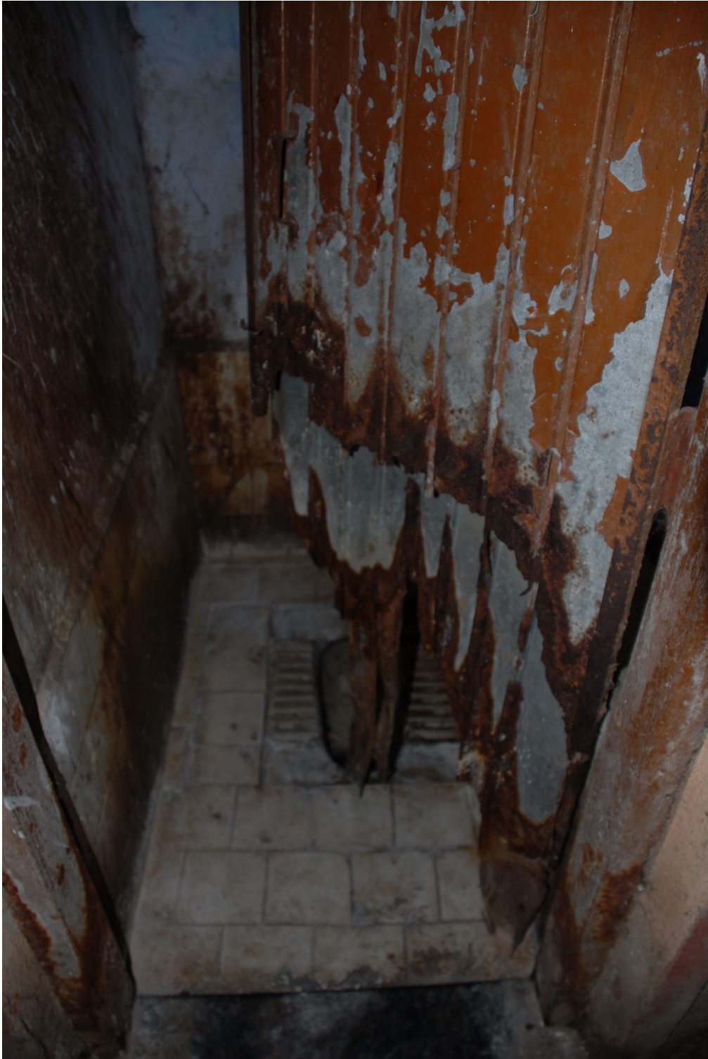
Figure 7.6 Toilet stall in Part I toilet block Credit: Author
