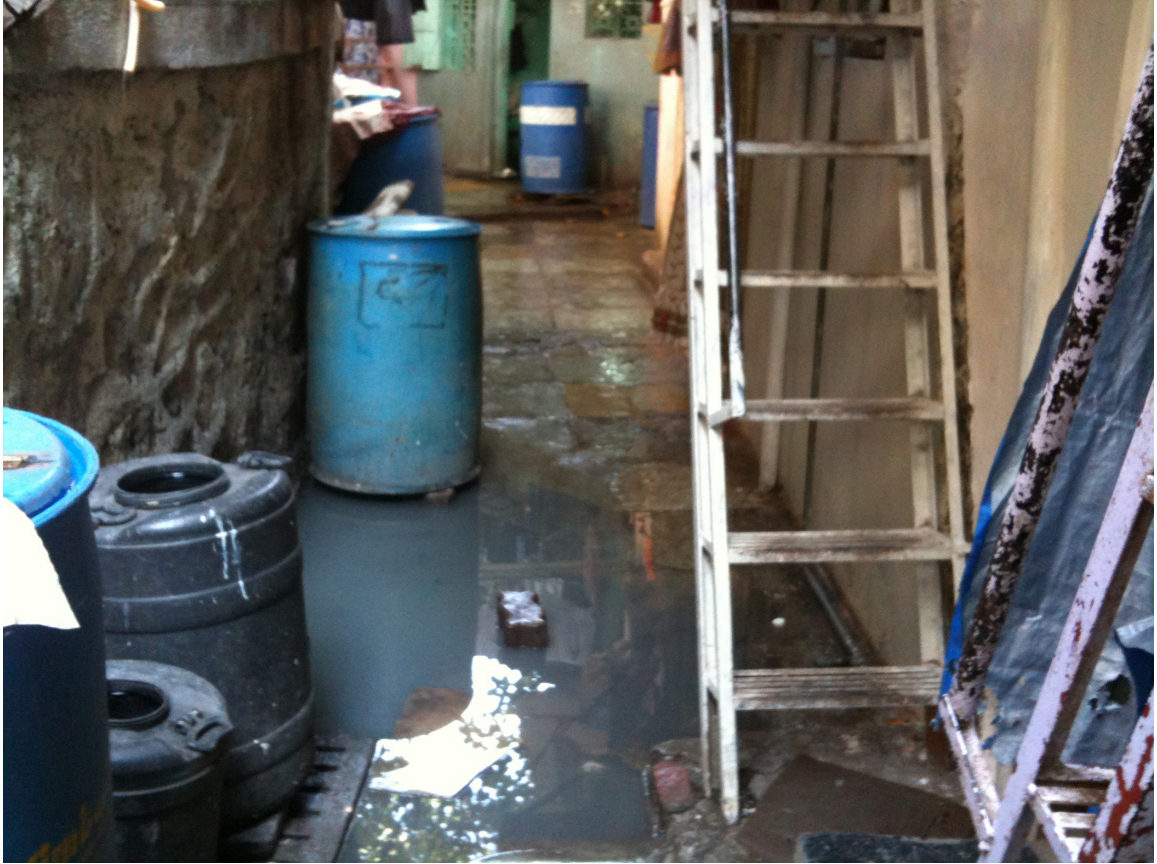
Figure 7.3 Flooding after a light rain Credit: Author
