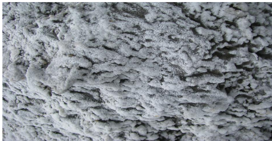
Figure 3.5: (a) Upper slopes of Oldoinyo Lengai with large rock structures locally known as the “Pearly Gates”. The photograph shows white covering of slopes representing weathered volcanic ash from the latest eruption; (b) close up of the carbonate effervescence present on the surfaces of the rain gullies on the upper slopes of the volcano. Photo courtesy of Matt Genge.
