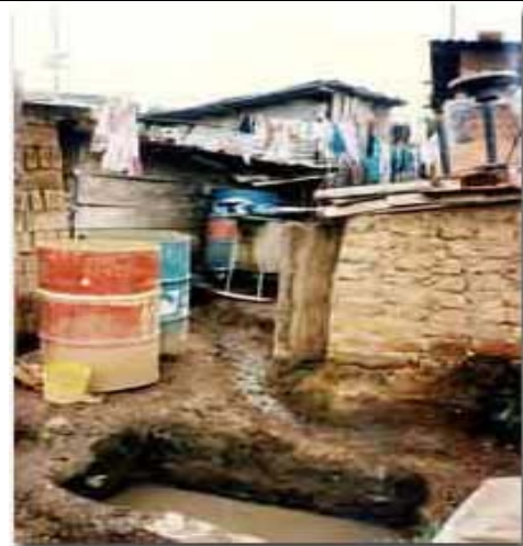
No access to clean water or sewage system (Bogota)
