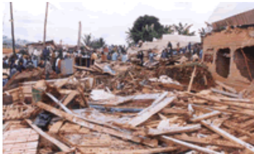
Demolition of informal settlements in a student residential area (Bonamoussadi, Yaoundé 06/10/02)
