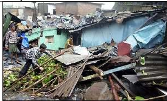
Informal settlements are subject to demolition (Bombay)
