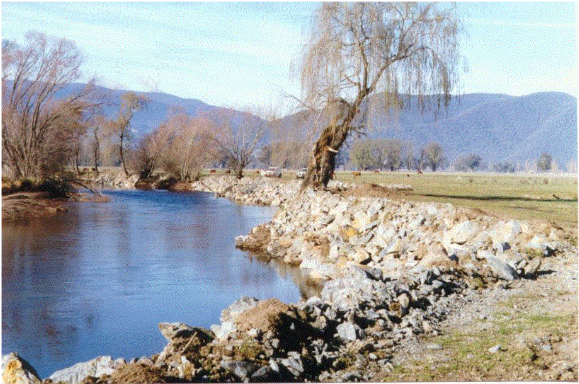
Figure 10 Example of bank recently rocked for erosion control, 1996
