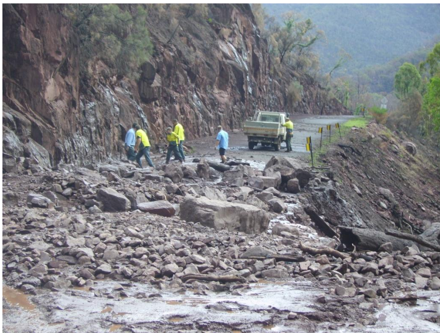
Figure 2. Debris flow event across Mt Tamboritha Road, near Licola in 2007. The town was closed off due to the road damage caused by the debris flow. Photo: Adrian Murphy
