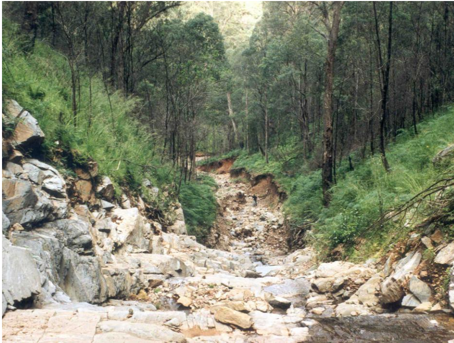
Figure 1. Channel scour after a debris flow event at Dingo Creek in the upper Buckland River, 2003. A fire fighter died after being caught at a road crossing. Photo: Gary Sheridan
