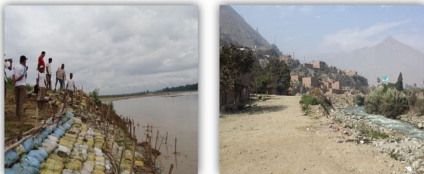
Fig. 17.3 Flood risk context in the Karnali river basin in Nepal (left panel) and the Rimac river valley in Peru (right panel). Photo Sources Practical Action and A. Keating
