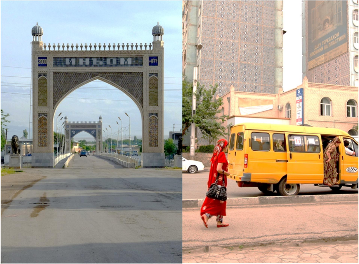
Illustration 18: The Amon bridge, the newest bridge over the Syrdarya
