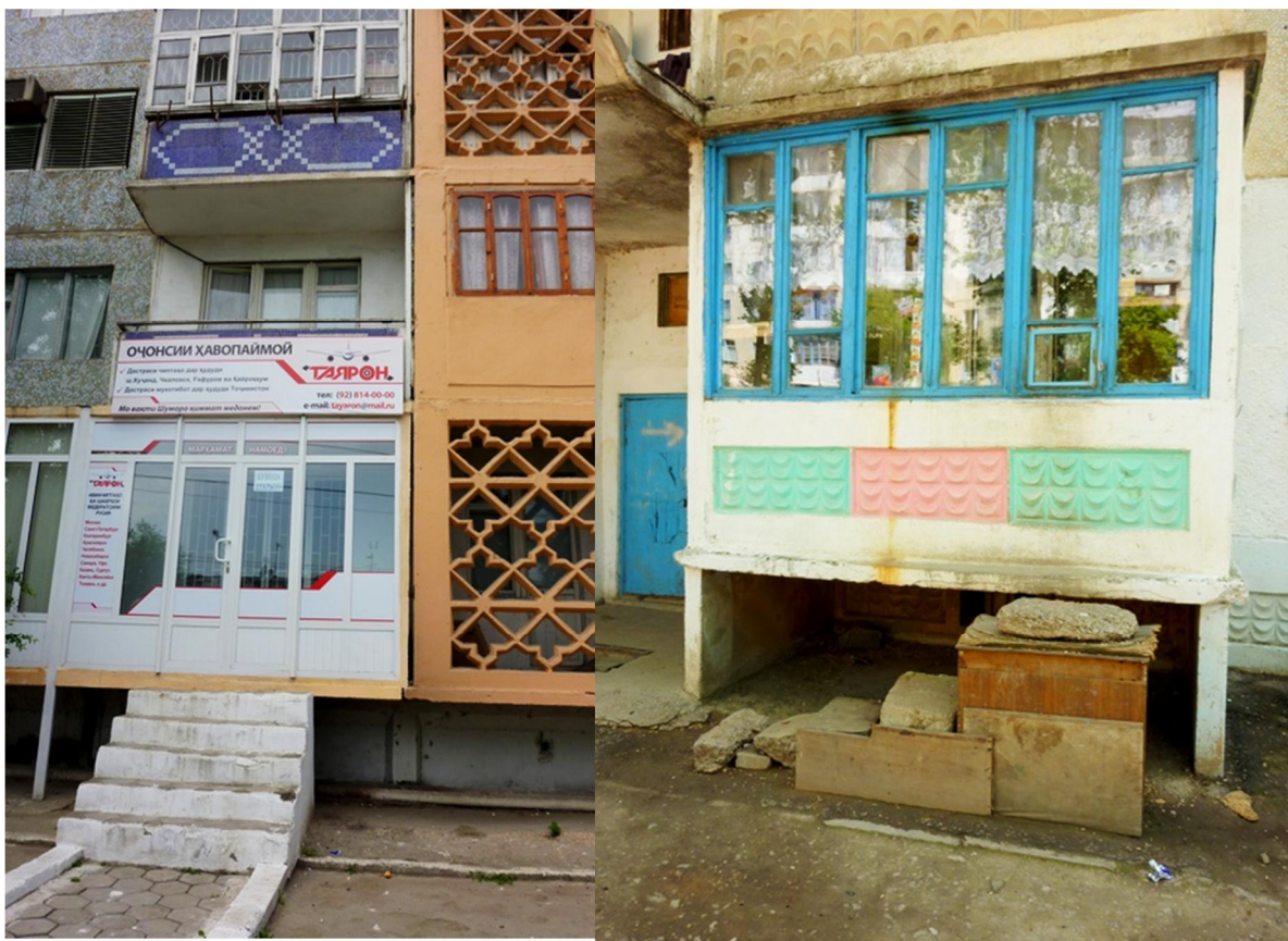
Illustration 48: New access to an office on the first floor
