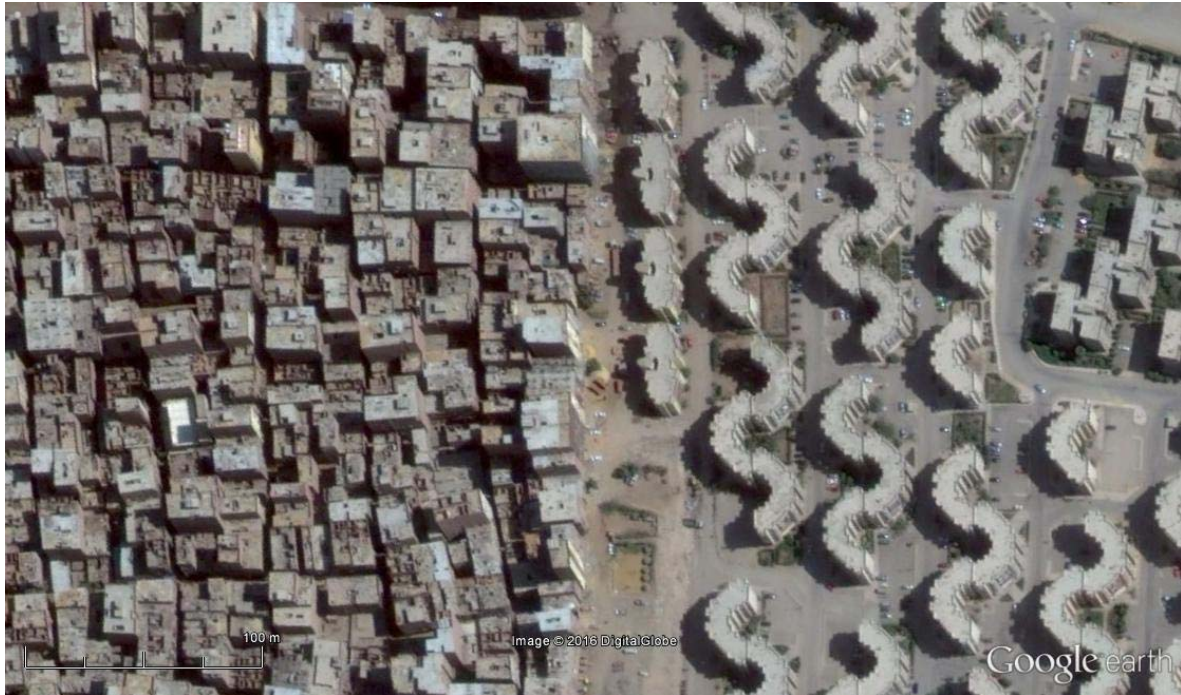
Figure 18: Part of Haggana (left) and an adjacent formal residential area (right).
