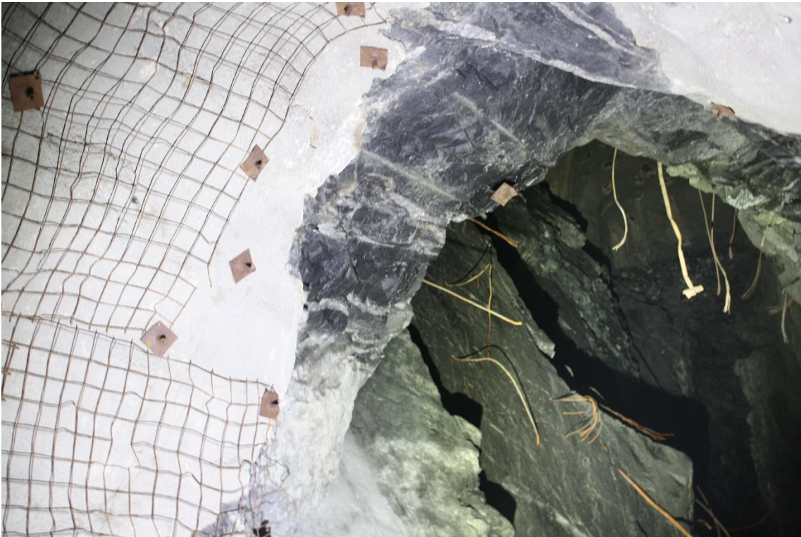
100A22 Footwall fault plane between rings 11-15 (on the right of the picture) next to the pillar (left) as described in section 6.5
