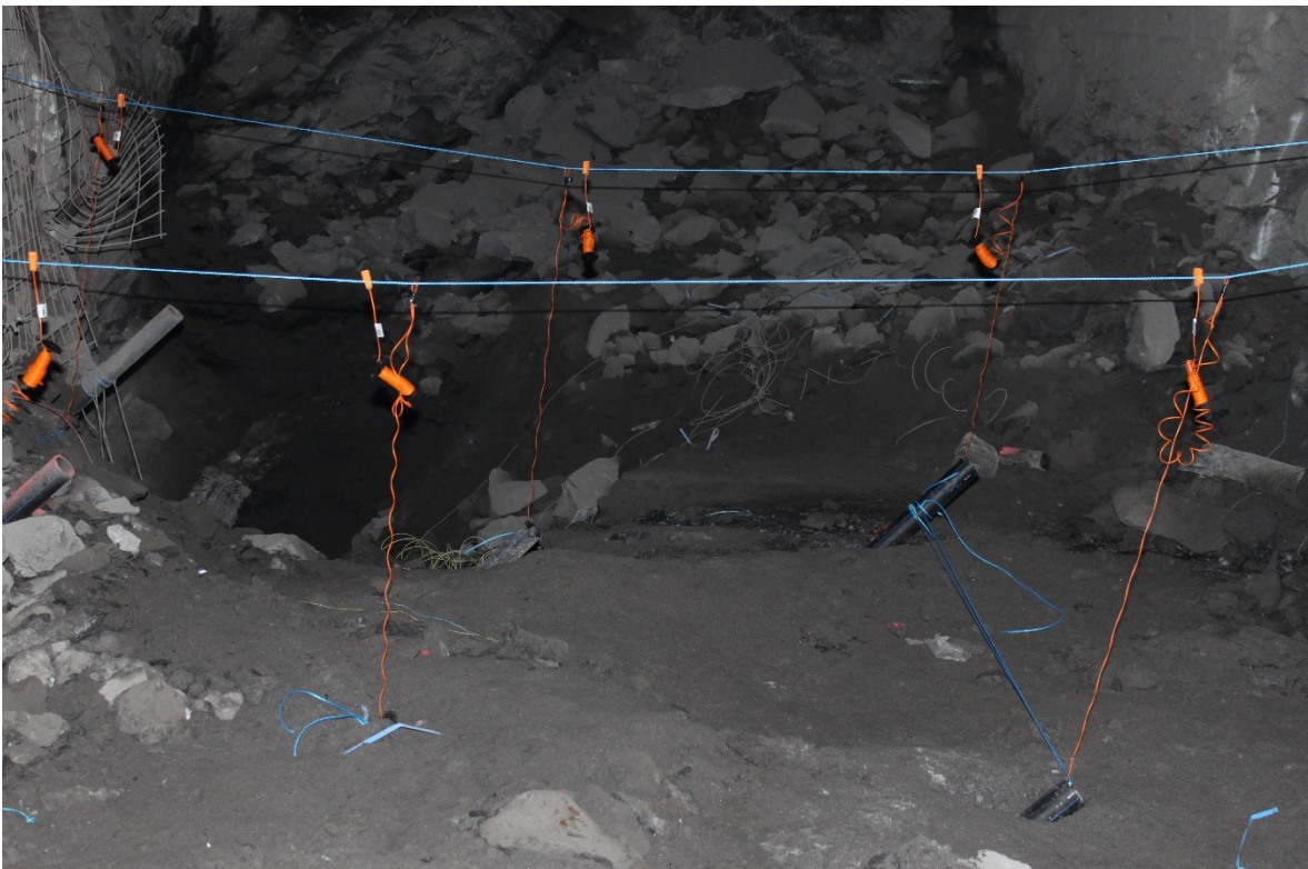
320K14 Stope rings 4-5 charged holes with programmed electronic detonators in place.
