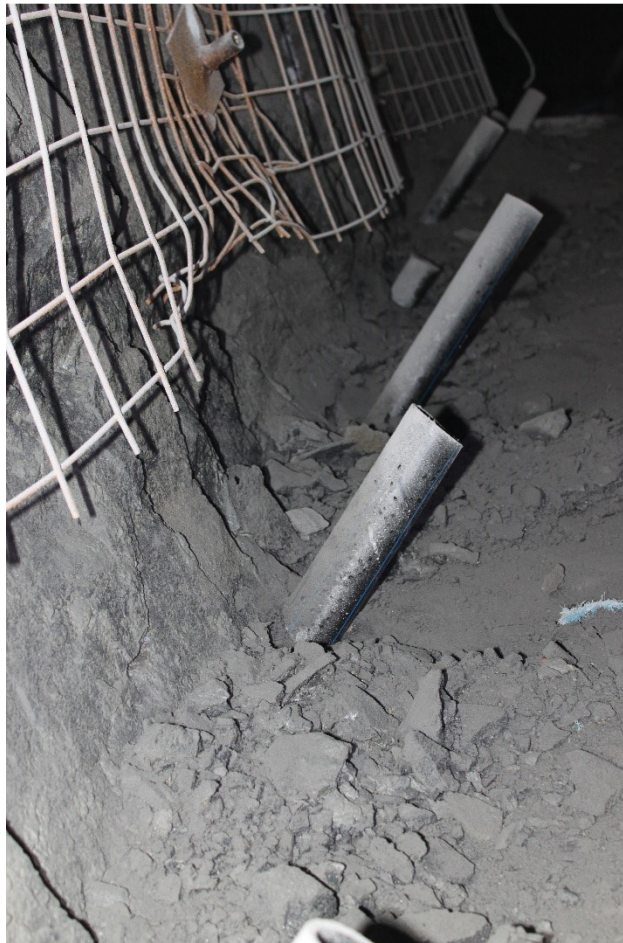
Figure 5.8: Polyethylene tubes installed at drillhole collars.
