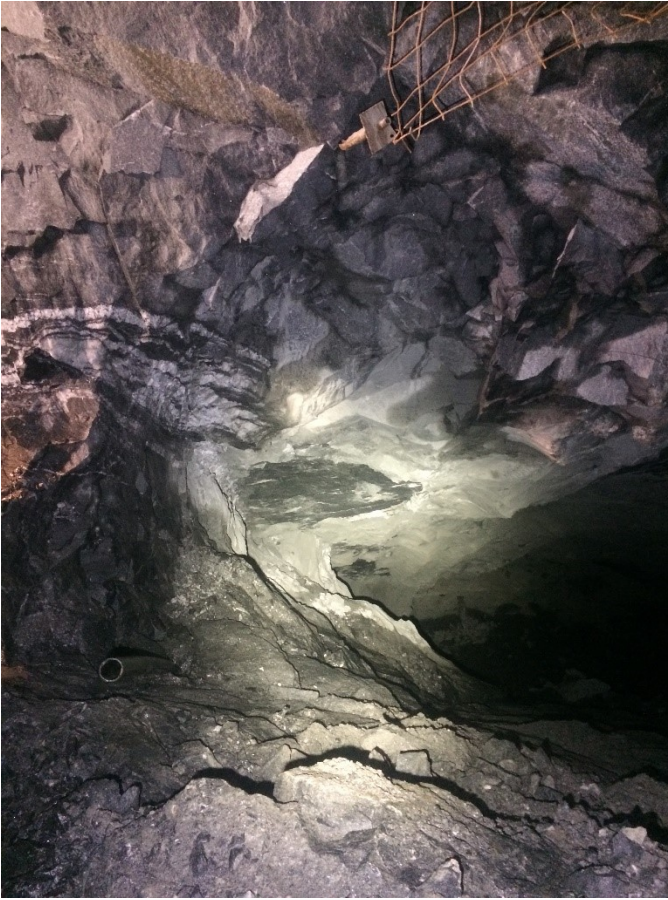
Failed detonation of footwall hole in 320K14 ring 15 as described in section 6.3.
