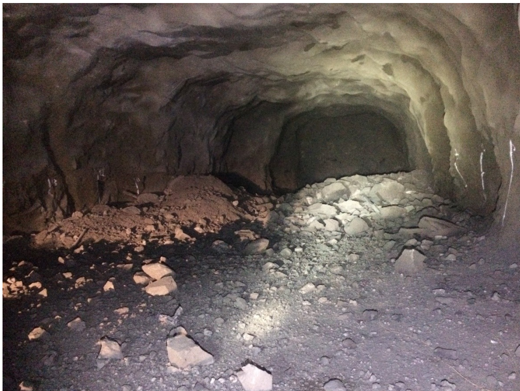
Figure 6.13: 80LpA22 Drift after blasting of rings 1-6.
