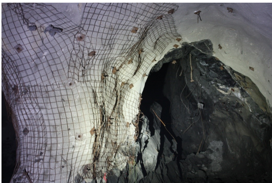
Figure 6.10: 100A22 Pillar after the stope has been mined out.
