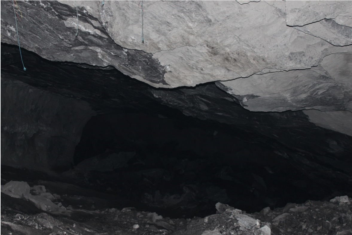
Figure 6.1: 320K14 Exposed surface (black) after hangingwall collapse rings 1-7.
