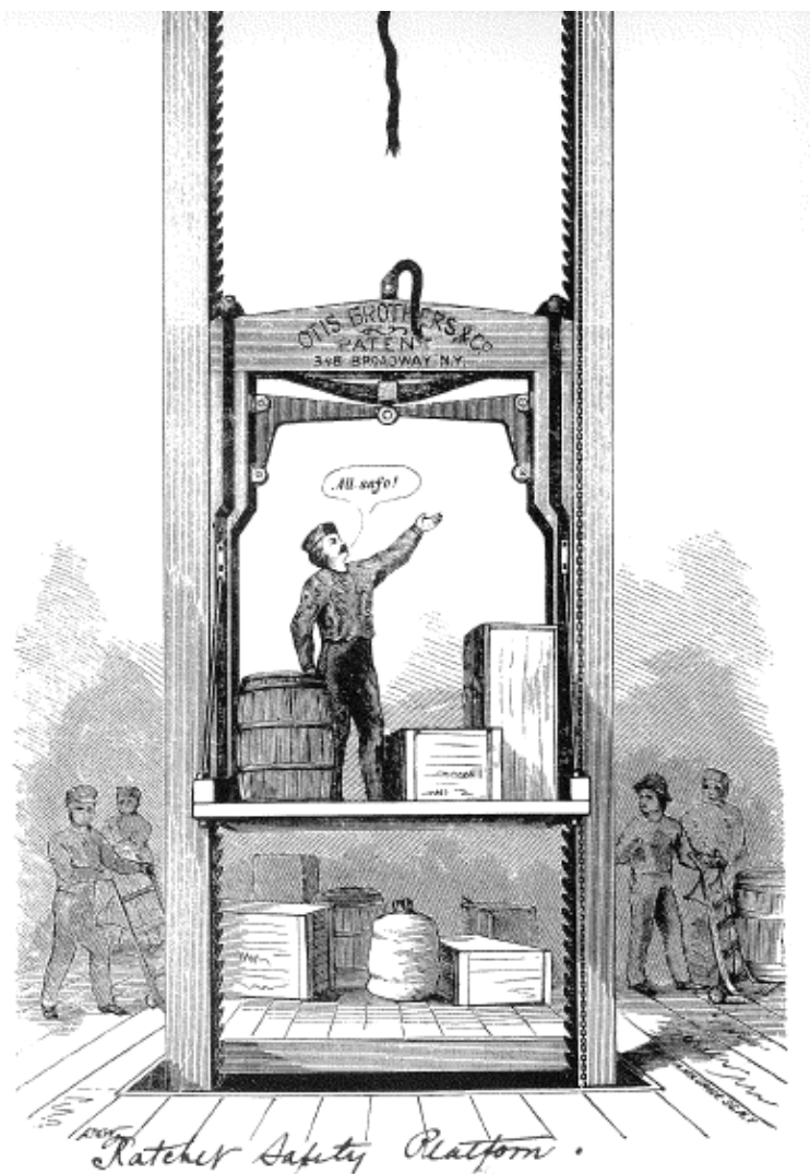
Figure 2. Demonstration of first automatic braking mechanism [8]
