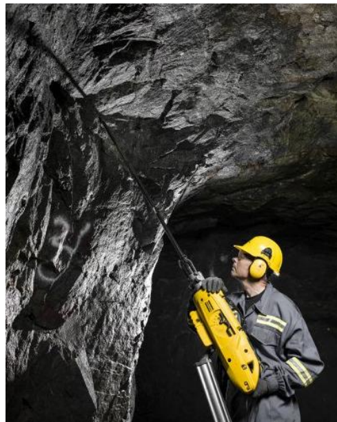
Figure 18. Handheld hydraulic rock drilling (AtlasCopco, 2014).
