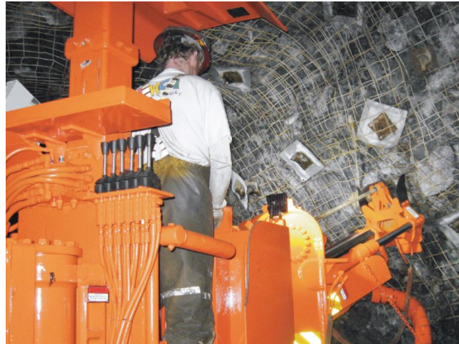
Figure 19. Semi mechanized bolt installation (Kendall, 2015).
