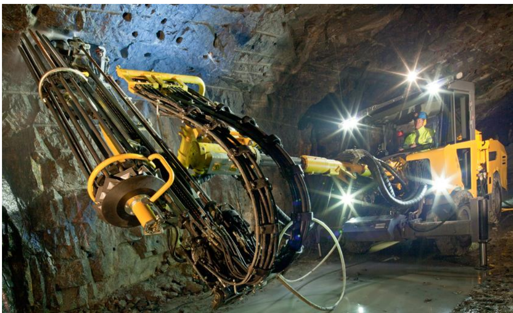
Figure 20. Fully mechanized bolt installation with the Boltec S (AtlasCopco, 2013).
