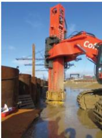
Figure 5-5: The RIC equipment working at site [11]
