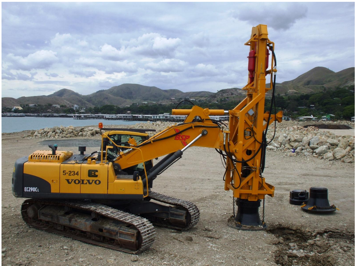
Figure 4-3: Rapid impact compactor on a track-mounted excavator [7]
