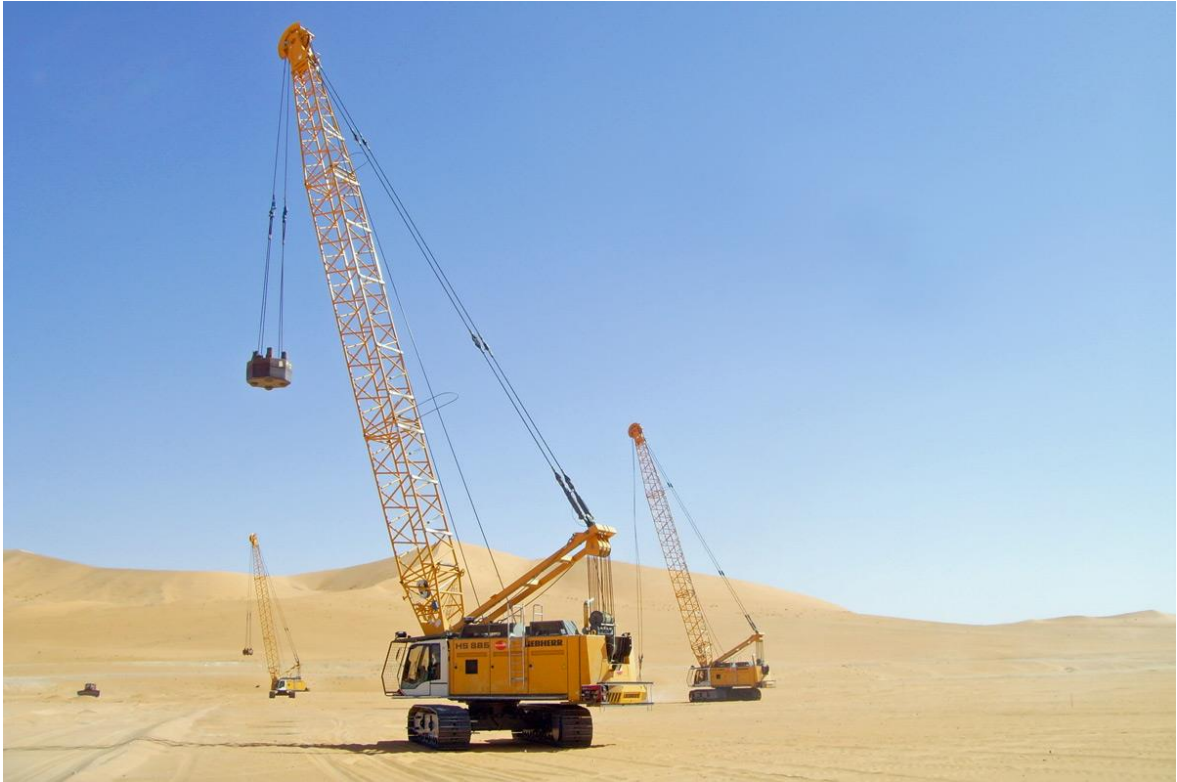
Figure 4-1: A crawler crane equipped with a free-falling weight [5]
