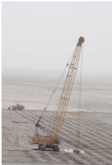
Figure 5-8: The both devices in action at the site a) Dynamic compaction b) Rapid impact compaction [12]
