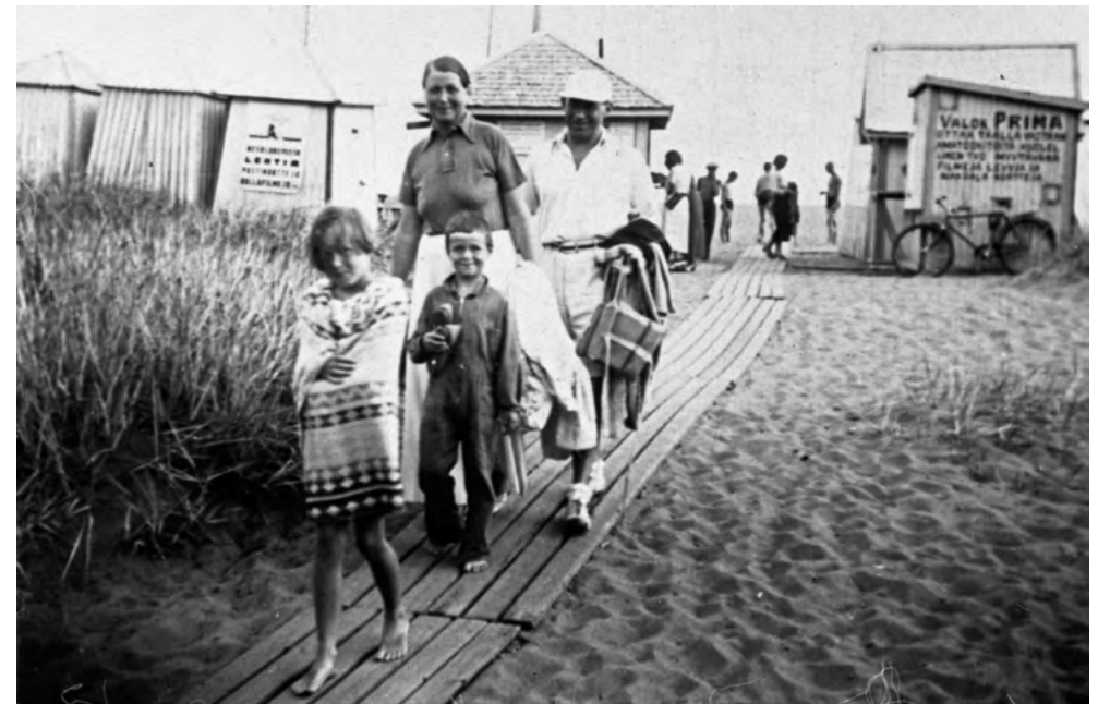
Fig. 71. The Aalto family spent the summer of 1934 at Terijoki on the Karelian Isthmus, making it possible to supervise the construction of the library. (AF)
