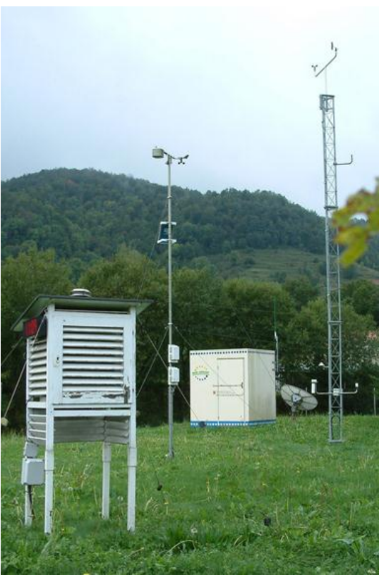
Weather station. Note the two anemometers set at different heights, the shelter housing the thermometer. (Sant Pau de Segúries, Spain). Photo: CEA Alt Ter – www.alt-ter.org
