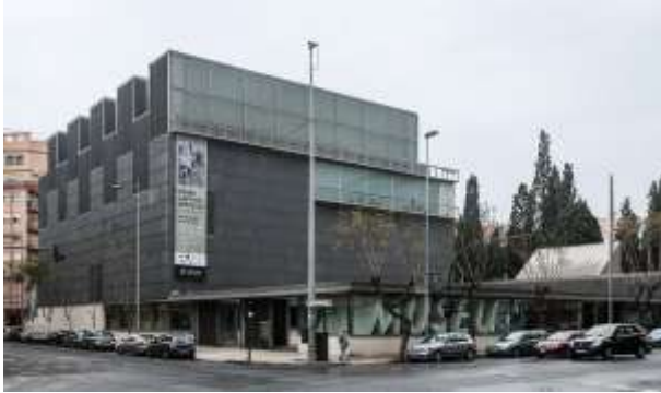
Fig. 1: View of the main volume of the building taken from the northeast.
