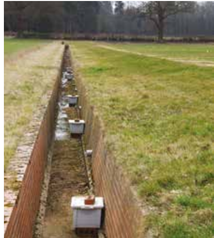
Drain outlets at eastern end of Broadbalk, 2010
