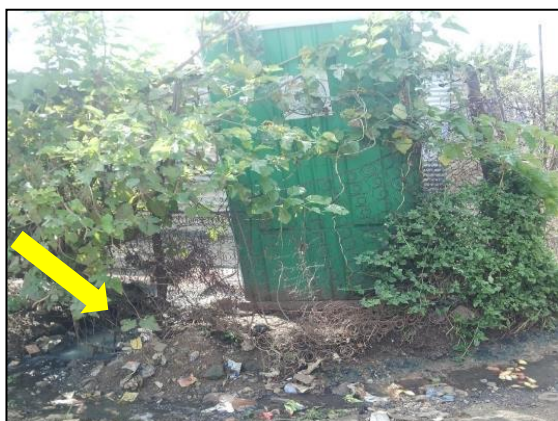
Figure 26: Over flowing mobile toilet (Source-research data)
