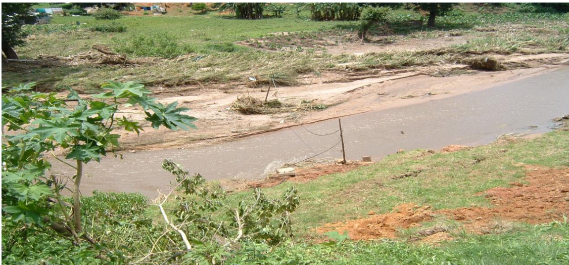
Photograph 3.6: Dangerous, exposed and sagging unauthorised electrical connection cable extending over a river in Umzinto, KwaZulu-Natal, South Africa 10
