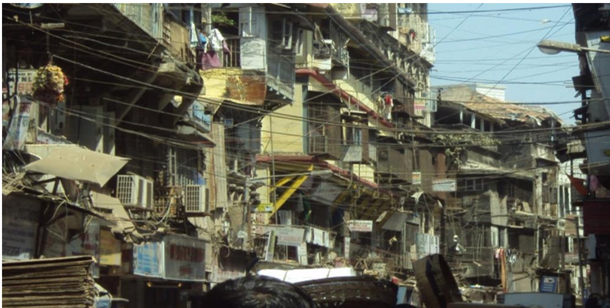
Photograph 3.1: Unauthorised electrical connections in a market area situated in Chennai, South India. 1
