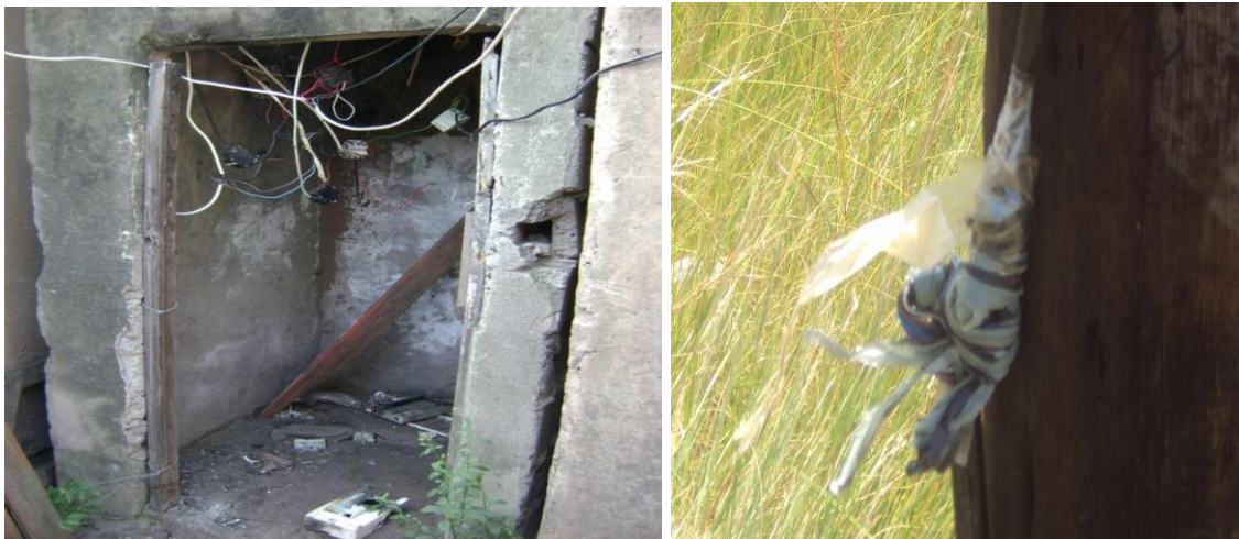
Photograph 3.9: Dangerous and exposed unauthorised electrical connections in a “switch room” and sealed with plastic in Jozini, Northern, KwaZulu-Natal, South Africa 13
