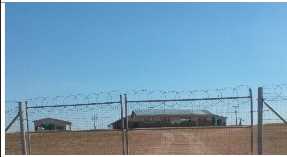
Photo 8: Fence around one of the schools
