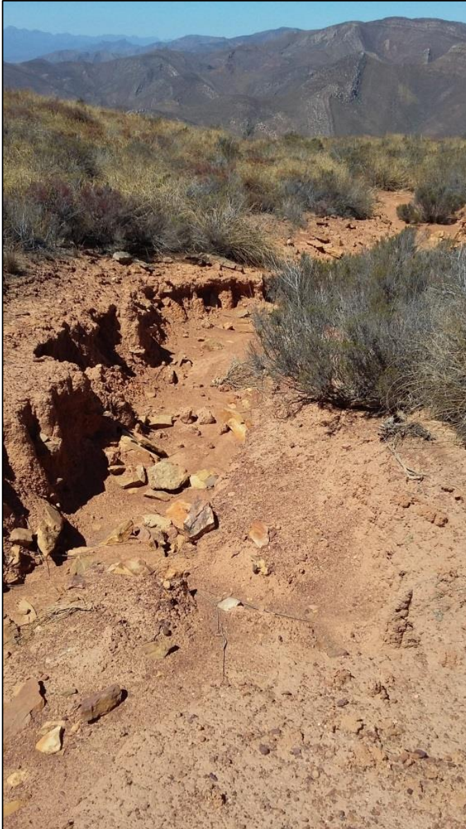
Figure 4.35: The soils of Community 5 are prone to natural erosion.
