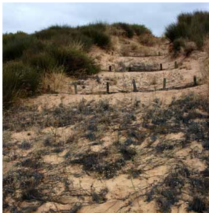
ABOVE: The covering of packed brush-bundles and in-between mulch on a bare track with pioneer vegetation establishing after the first rehabilitation attempt.
