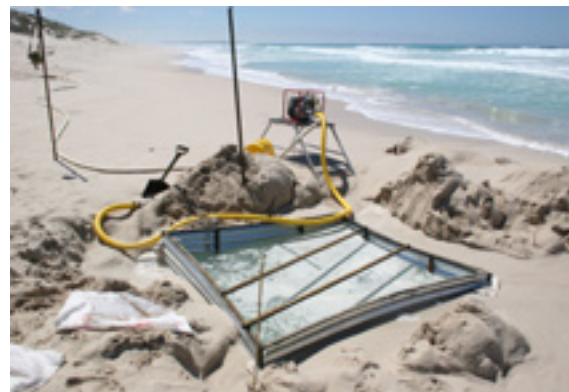
Figure 25: Corrugated iron cofferdam.
