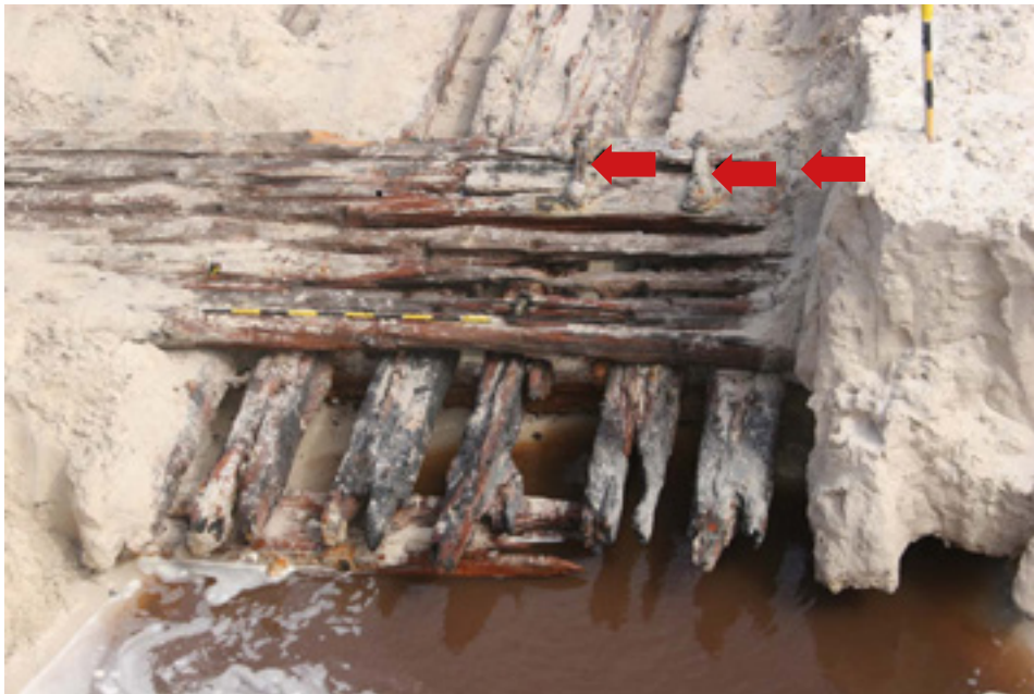
Figure 39: Preventer plates indicated by red arrows.
