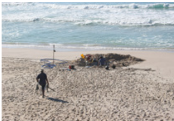
Figure 26: Digging inside cofferdam.
