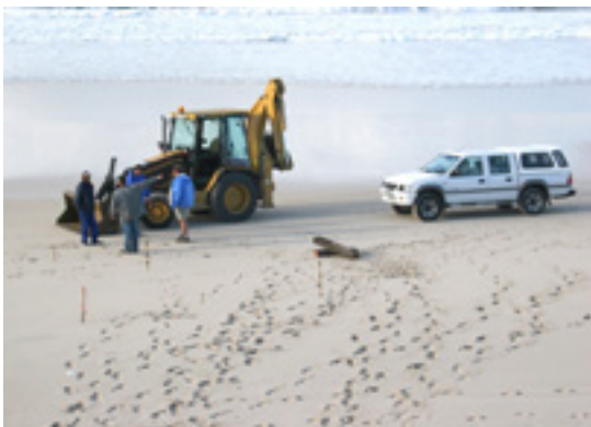
Figure 28: Digger/Backhoe on Meermin Site 1.
