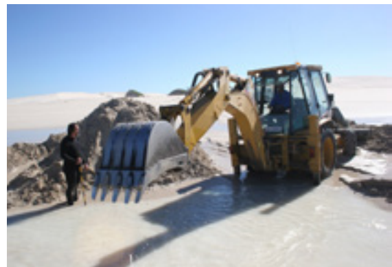
Figure 29: Incoming tide makes it impossible to continue with the Digger/Backhoe.
