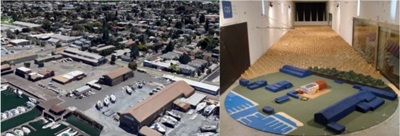
Figure 6 – Aerial view (left), wind tunnel model of the main building and surrounding buildings (right)
