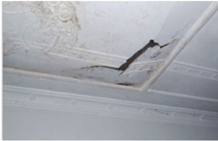
Fig. 2. Damaged Ceilings and Mould growth with Leaking Roofs – (modified [9])
