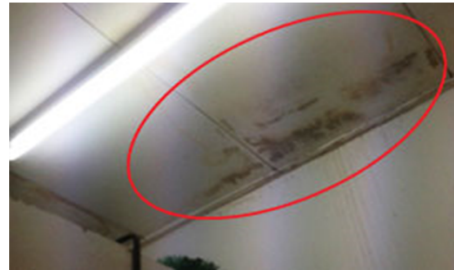
Fig. 2. Damaged Ceilings and Mould growth with Leaking Roofs – (modified [9])
