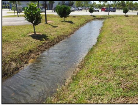
Figure 1: Wet grassed swale
