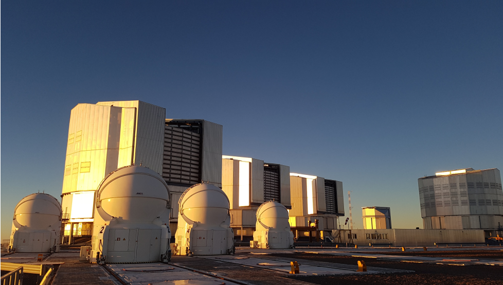
Figure 3.1: The four Unit-Telescopes, that are about to open, and the smaller Auxiliary-Telescopes. In the back between UT3 and UT4, the VLT Survey Telescope is visible.
