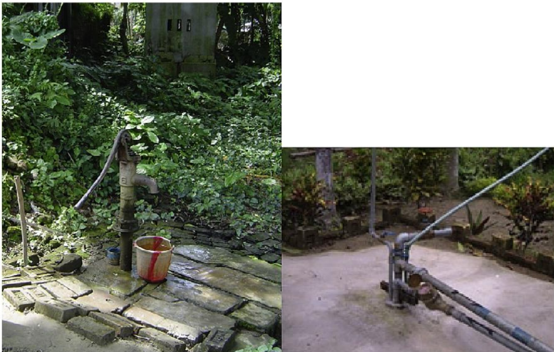
Fig. 4. A view of the site before and after installation of the treatment plant.
