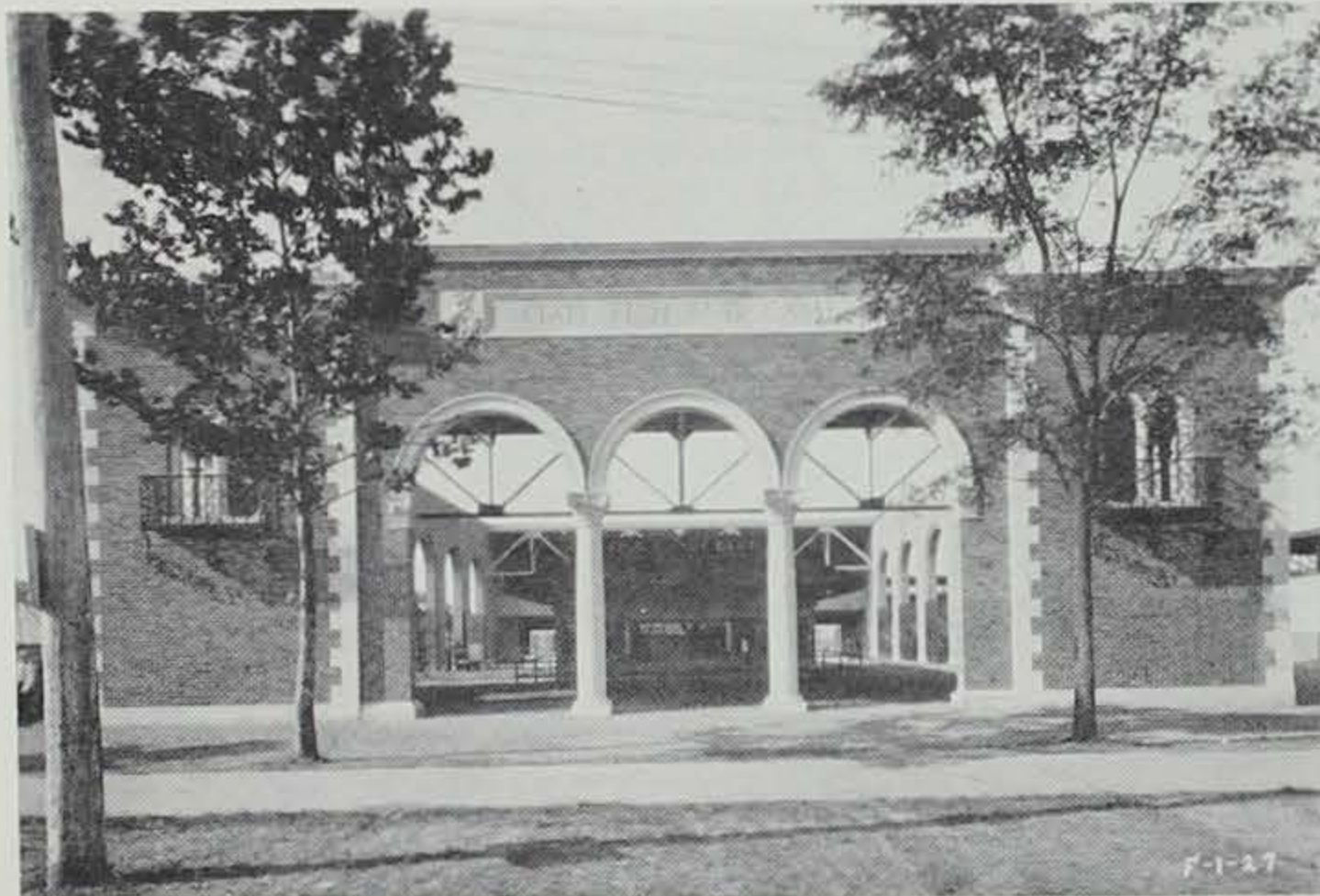
The 1923 Fair started before the roof over the new exhibit building was completed.
