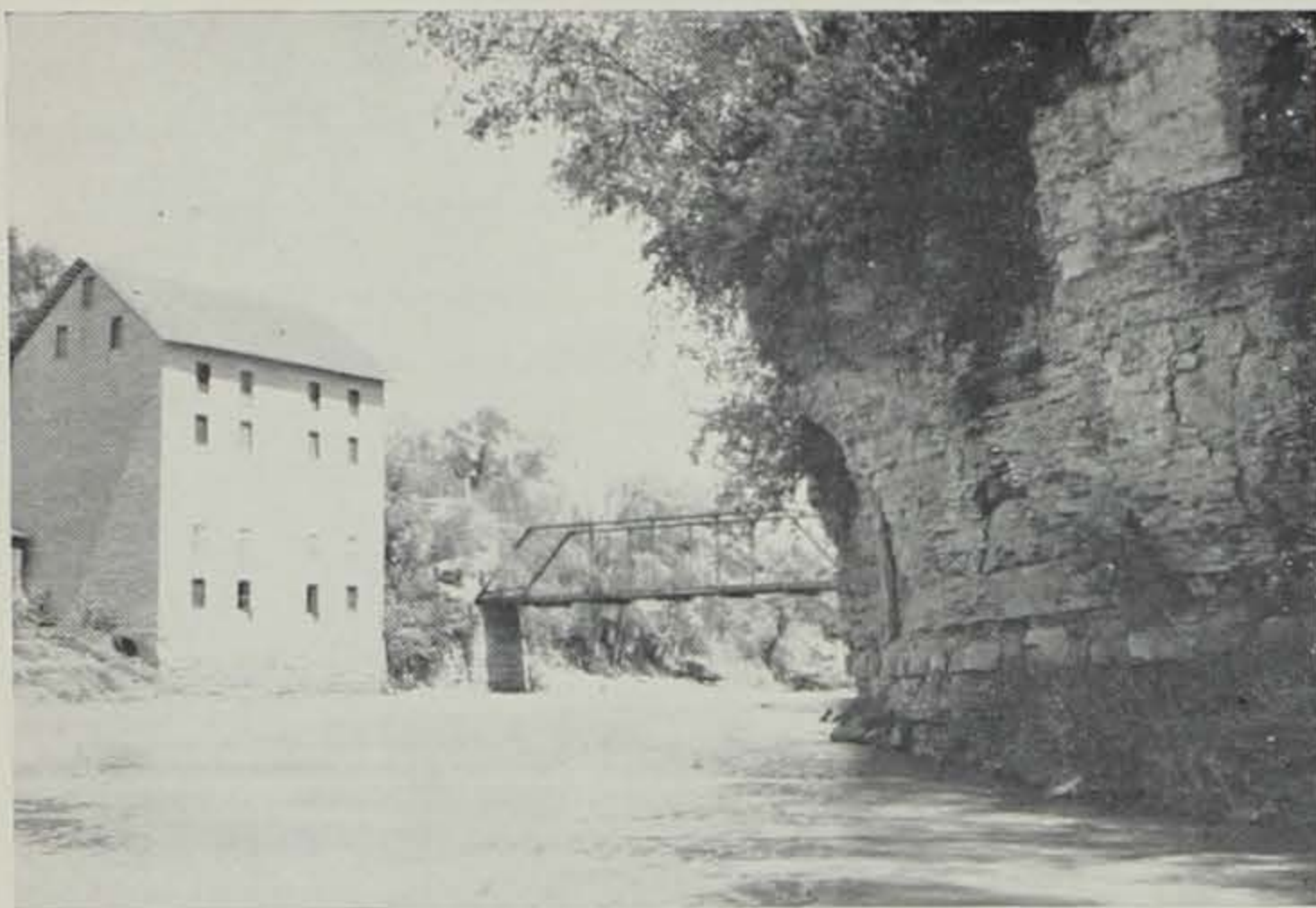
Like part of the limestone bluffs, the old Motor grist mill has stood beside the swift Turkey River for nearly 100 years. Church and Allen Photo.
