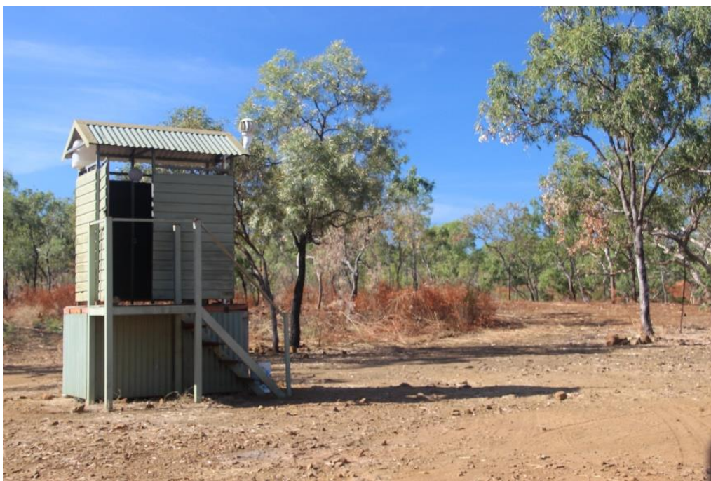
Figure 3.7: Walsh Point campground has one unmaintained toilet which is located in a large cleared area. (Image: author supplied).
