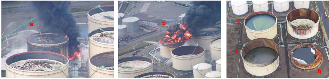
Figure 3-14 Tokachi-oki earthquake in 2003. From left to right: ring fire in a crude oil tank; open-top fire in a naphtha tank; sinking of floating roofs in two kerosene tanks
