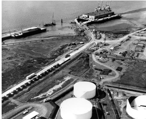
Figure 3-3. Anchorage, Alaska, 1964. Vibration and ground fractures damaged some structures in the port area, including the fuel tank seen in the lower right
