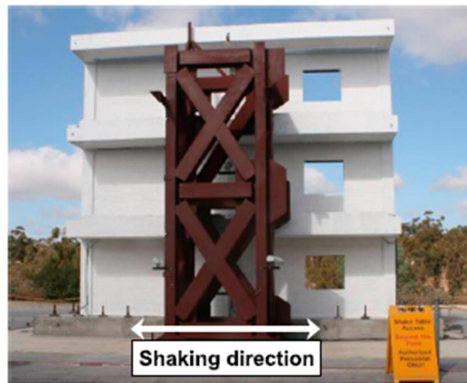
Figure 5.5: Front view of the specimen (from Moaveni et al., 2013).
