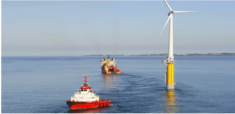
Figure 1.9: Hywind floating wind turbine, Statoil desing.
