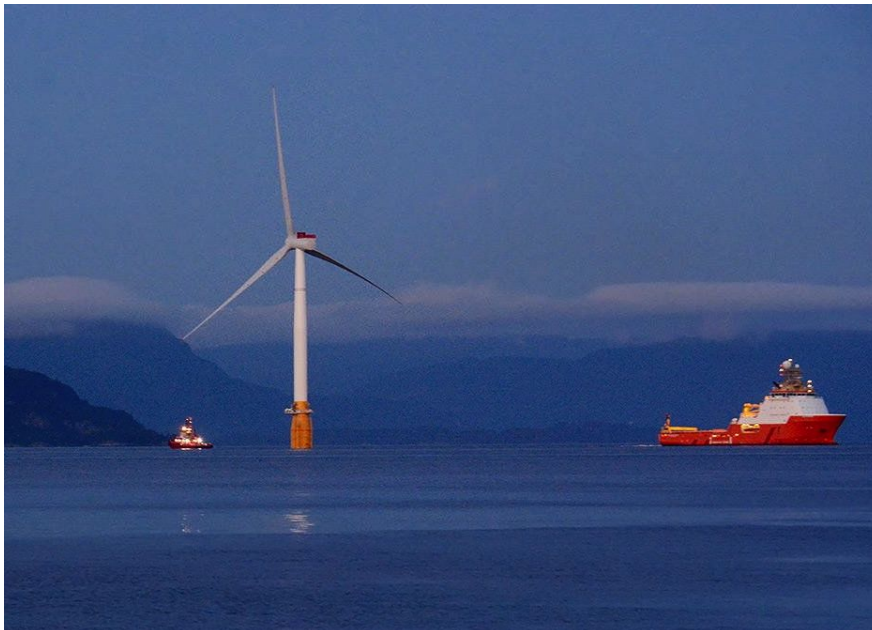
Figure 1.10: Hywind floating wind turbine, Statoil desing.
