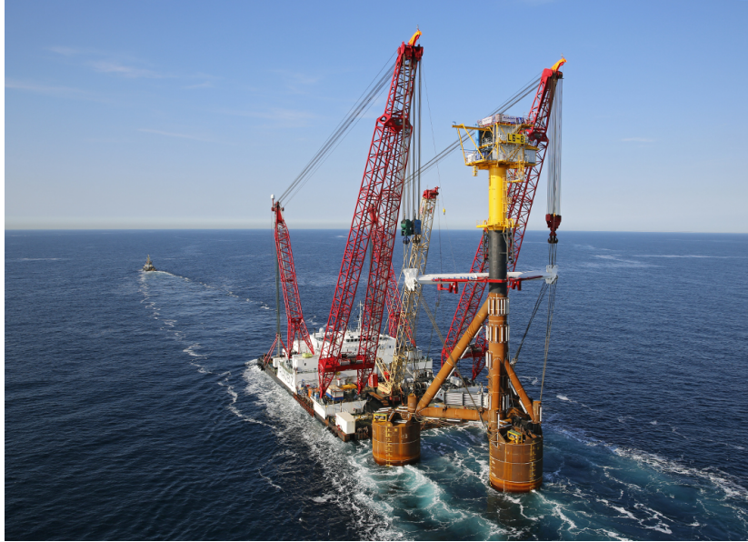
Figure 1.2: Transportation of Floating wind turbine foundation.
