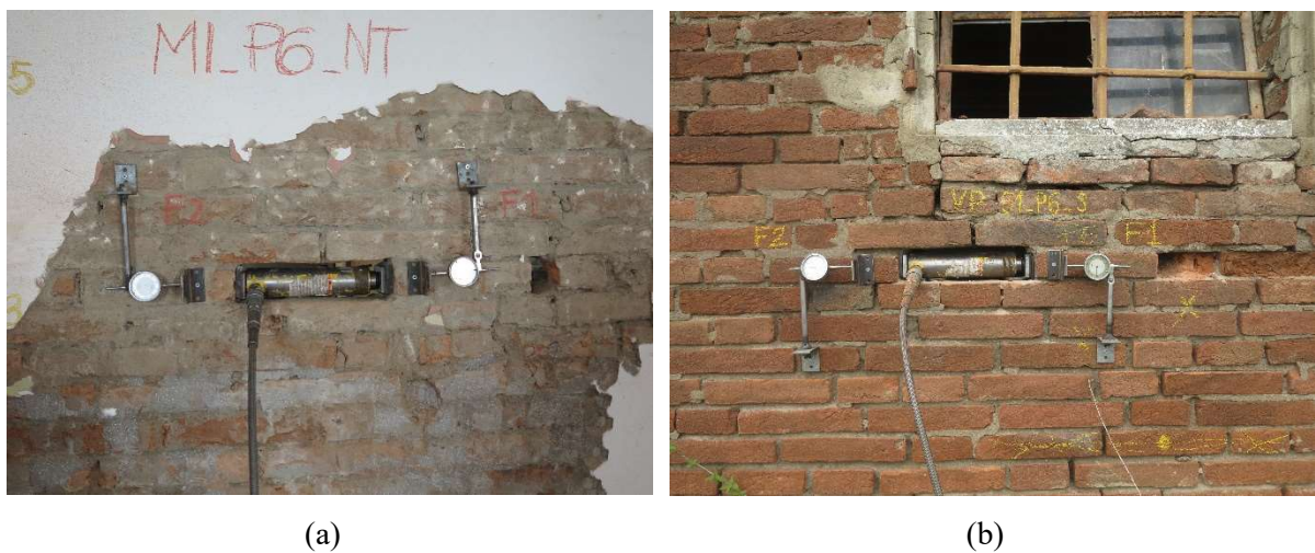
Figure 3.8. Shove test: (a) at ground floor (max vertical stress); (b) below window openings (zero vertical stress)
