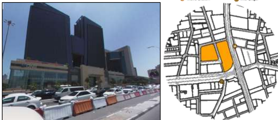
Fig-15: Traffic congestion amid construction
