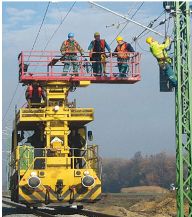
Figure 1.1 Overhead line's inspection in Hungary. (Innoteka, 2012)
