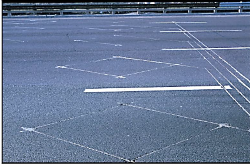
Figure 1.1: Road traffic monitoring via inductive loops. Example inductive loop configuration where a diamond-shaped loop is installed on each lane of the road. Source: [1].
