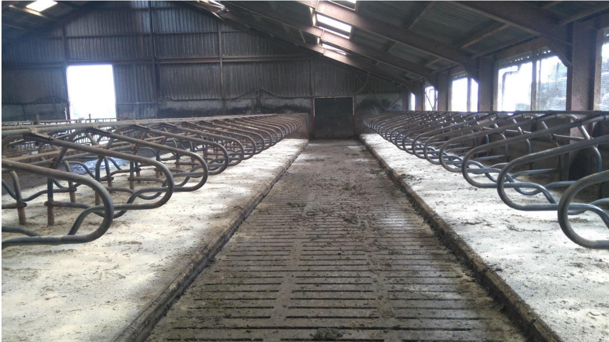
Figure 1: Example of the flat concrete free stalls topped with a rubber mat (it is white because of a thin layer of saw dust to absorb moisture) and a corridor with a slatted floor at Mts. Bosma
