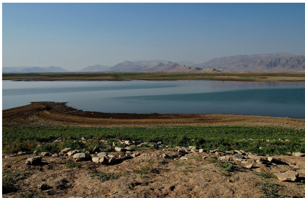
Figure 2: The Dokan Dam.
