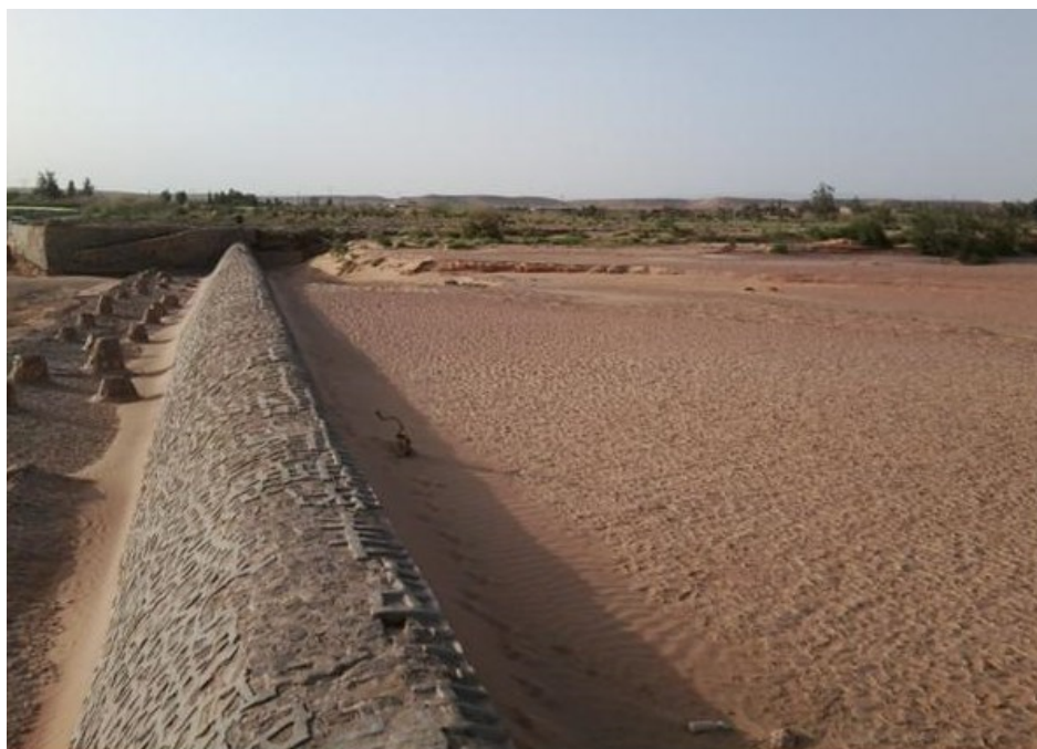
Fig. 8. Second New Greager Weir Dam (Photo. Authors, 2015)
