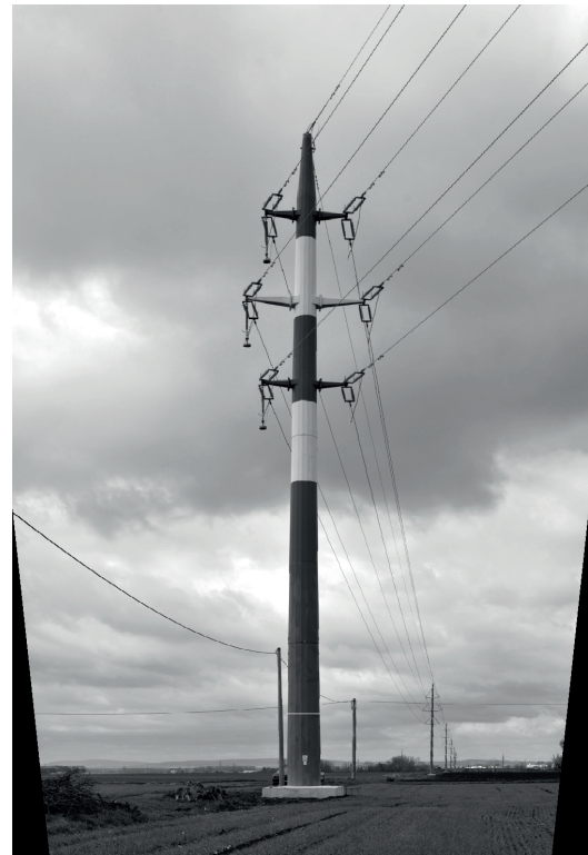
Fig. 1 Tilt of image by using perspective transformation (pylon 13).
