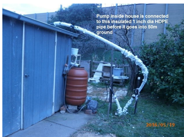
Figure 5: Top of 1" U-tube at East corner
