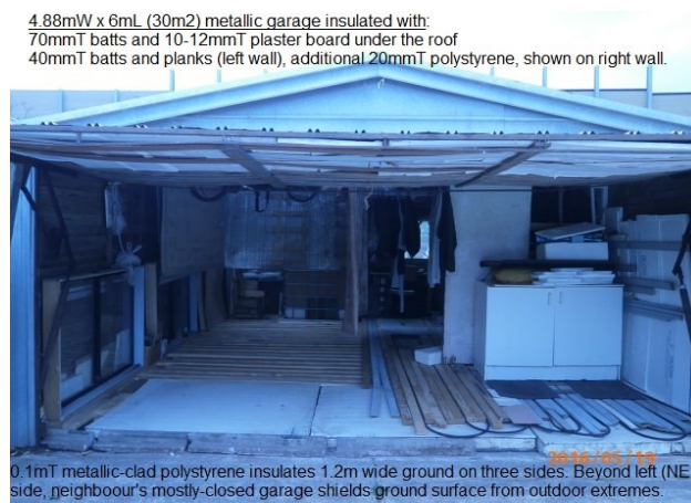
Figure 4: SW view of experimental building
