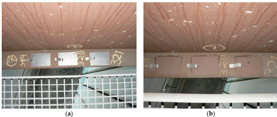
Figure 5. Corrosion samples on the upper surface of the bottom flange at the time of installation (a) and after 1 year of the exposure (b).
