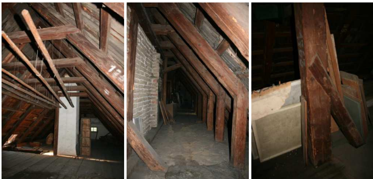
Fig. 2: The inner view of the truss.
